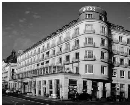
AMAG-Autohaus am Utoquai in Zürich 8
